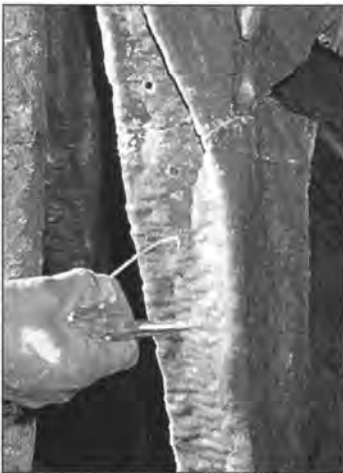
Figure 18. Install a stabilization pin if necessary and drill small holes above and below the break joint to accept supporting wires.
