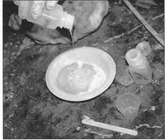
Figure 4. Mix archival-grade epoxy with crushed rock for filling cracks and seams.
