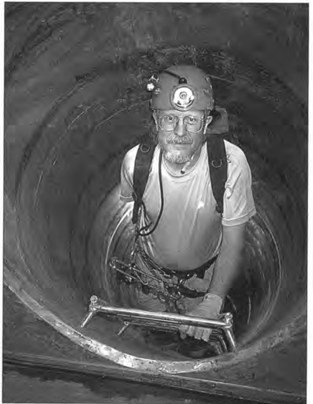
Figure 3. In 2002, the rusted culvert was replaced. A stainless steel culvert with an air lock entry was installed in Lechuguilla Cave. (See page 6 of color section.)
