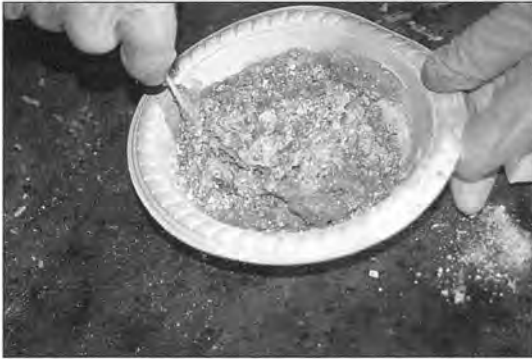
Figure 6. Mix drill dust or crushed rock with an approved epoxy to create color and a workable consistency for filling gaps and cracks.
