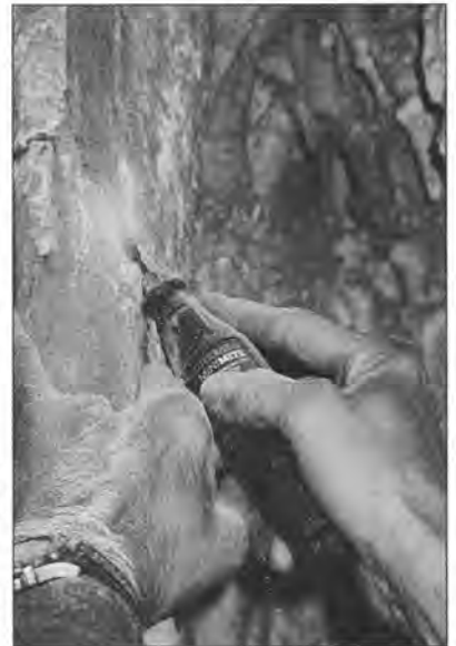
Figure 9. Try to blend, camouflage, or conceal the repair joints. Texture epoxied seams with a Dremel tool, sand paper, dental picks, drill dust, soil, or sand.
