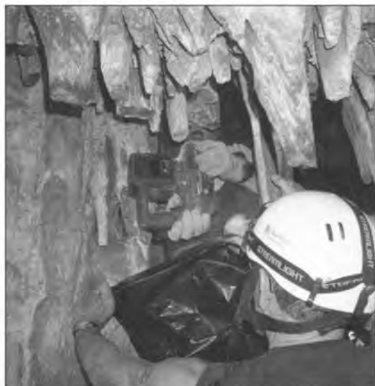
Figures 1 and 2. Large trash bags will easily capture most drill dust. If the powder is needed for filling cracks, gaps, or drill holes, capture and save it in a Ziploc.
