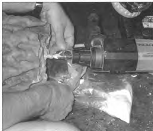
Figures 1 and 2. Large trash bags will easily capture most drill dust. If the powder is needed for filling cracks, gaps, or drill holes, capture and save it in a Ziploc.
