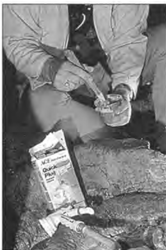
Figure 2. Quick-setting cement products are the recommended materials for reconstructing and sculpting broken rimstone dams.
