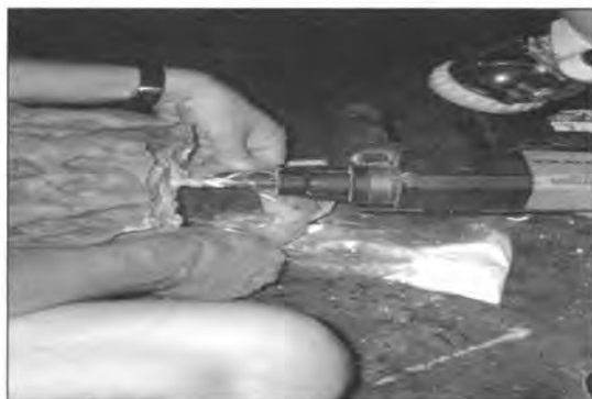
Figure 4. Toothbrushes are good tools to carry in speleothem repair kits. Use a toothbrush to clear the drill dust from large drill holes and to aid in the final cleanup of repair sites.
