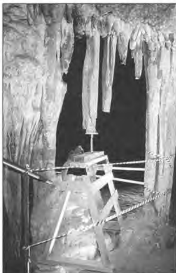
Figure 6a (before) and Figure 6b (midway through repair). These two photos show the reattachment of the upper piece to the ceiling. In the second image, the support jack is cordoned off for safety and left in place for several weeks to assure proper curing of the archival epoxy.
