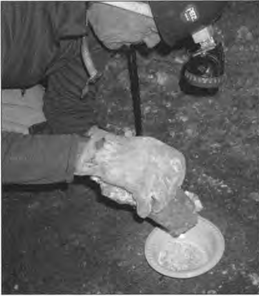
Figure 4. Mix archival-grade epoxy with crushed rock for filling cracks and seams.
