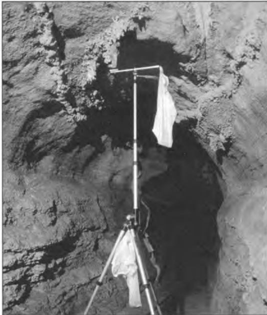
Figure 4. For overhead repairs in tall passages, extend the center tripod leg vertically from the lower fulcrum. Create an upper fulcrum with a mini tripod head and short padded crossbar.
