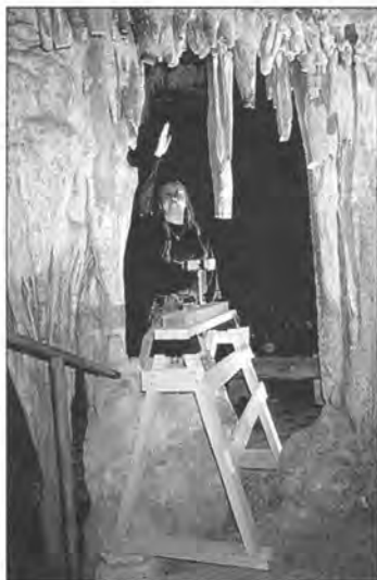
Figure 6a (before) and Figure 6b (midway through repair). These two photos show the reattachment of the upper piece to the ceiling. In the second image, the support jack is cordoned off for safety and left in place for several weeks to assure proper curing of the archival epoxy.
