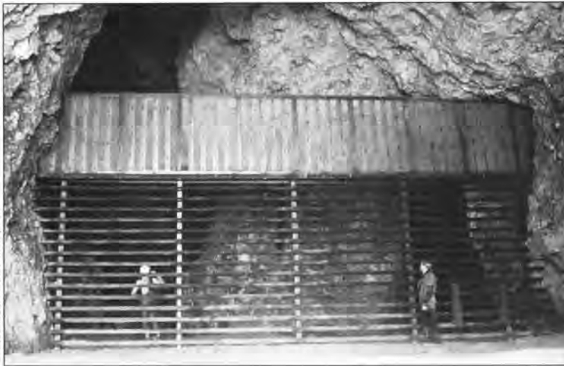
Figure 9. Half or “flyover” gate. Note the removable bar at bottom right. Expanded metal mesh covers the overhanging top portion, making it extremely difficult to climb over. Coating the overhang with grease also helps repel trespassers.
