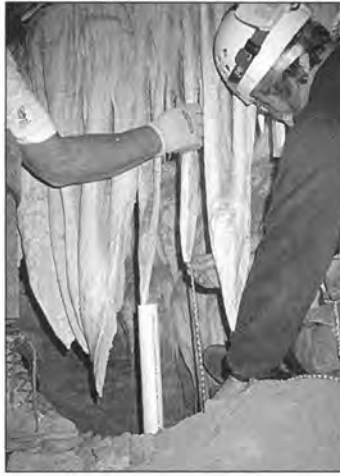
Figure 3. Measure the length needed for proper bracing and cut PVC pipe to size.
