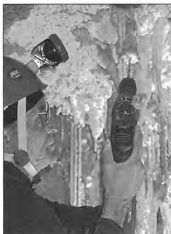
Figure 14. Drill the hole for a support pin in the top stal section that remains attached to the ceiling. Jim Werker is drilling to prepare a site for repair in Lower Cave, Carlsbad Caverns National Park, NM.
