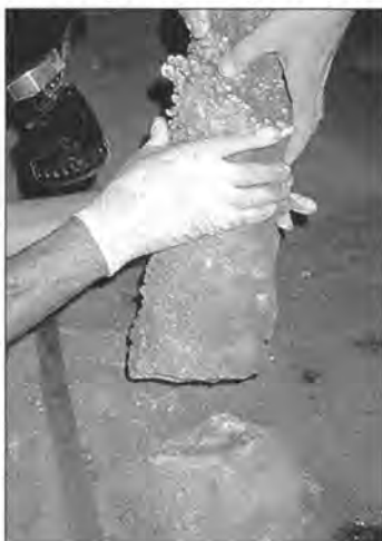
Figure 2. Click-fit the upper piece onto the base and allow several days for the epoxy to thoroughly cure.
