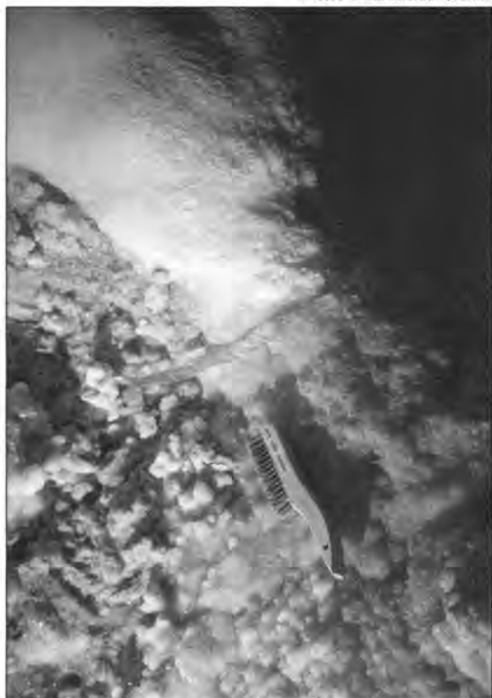
Figure 3 (before and after). Use a stainless steel brush to clean dense gypsum surfaces. The brush is sitting on soiled gypsum that is not yet restored.
