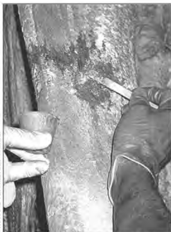
Figure 8. A mixture of rock dust and archival epoxy conceals the drill holes, grooves, and wire supports.
